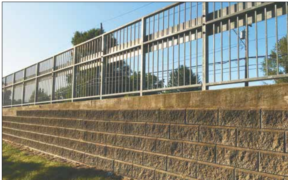
A cast-in-place wall was the design that most residents along Capitol Highway liked. Railings are required where a fall hazard is present. Residents preferred railing that was painted black, which is designed to fade into the landscape. (Post photo by Erik Vidstrand)
