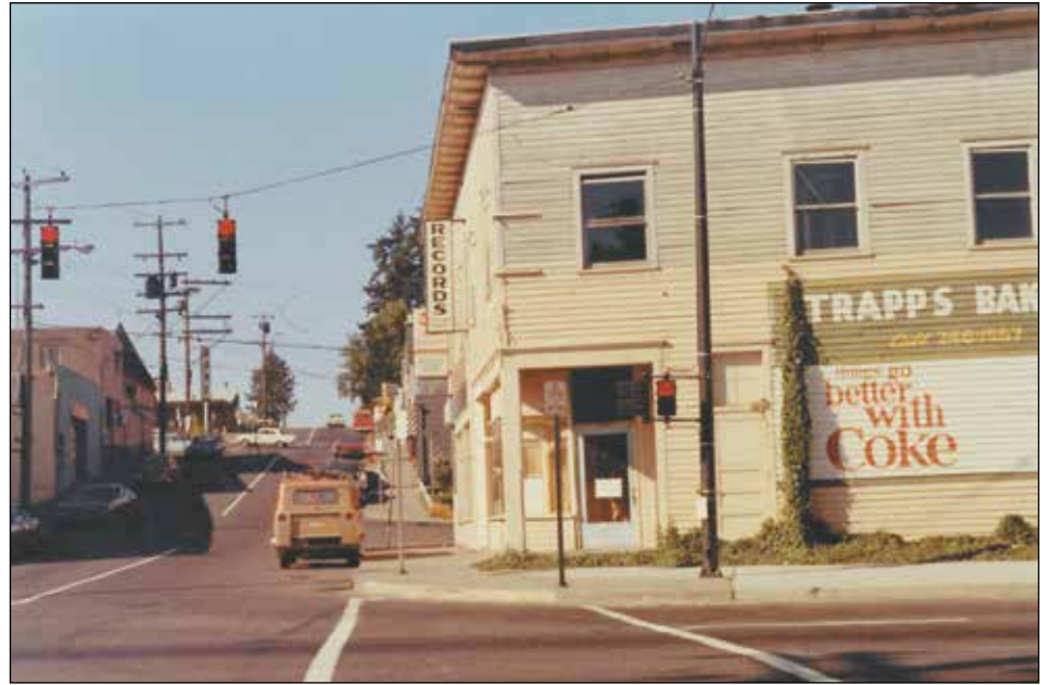
A photo taken circa 1970 of the historic Nelson Thomas building in Multnomah Village. (photo courtesy of Dan Bixel)
