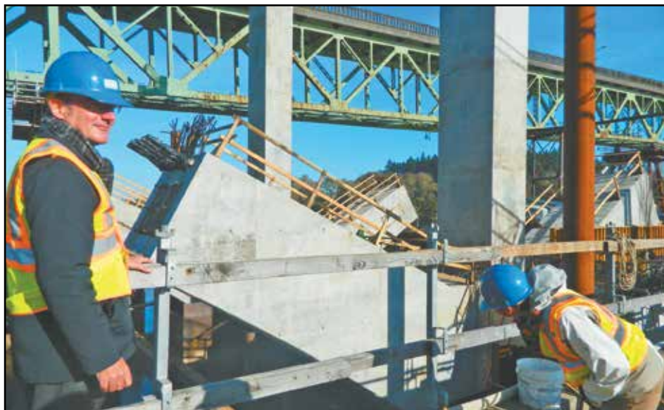
Mike Pullen (left), spokesman for Multnomah County, stands in front of angel wing support structure for the new steel arch spans being manufactured in Washington. (Post photo by Erik Vidstrand)
