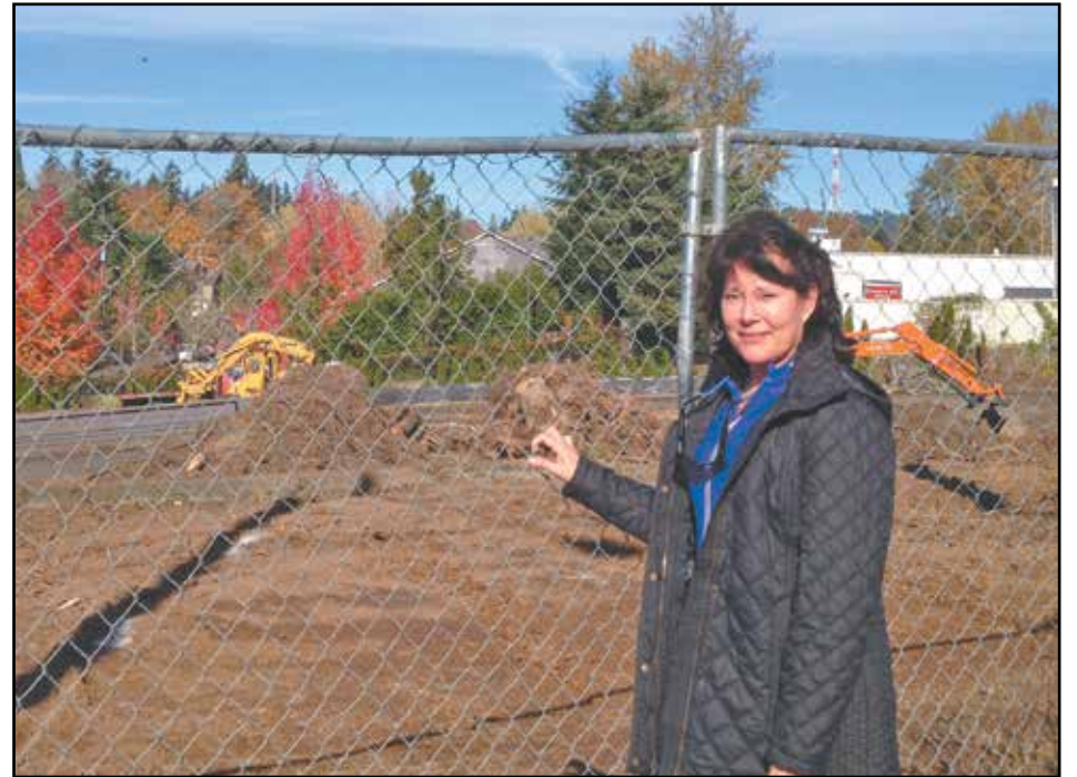
Nancy Craig of Multnomah inspects the Fred Meyer fuel center construction site on Southwest 24th Avenue near Barbur Boulevard. (Post photo by Erik Vidstrand)
