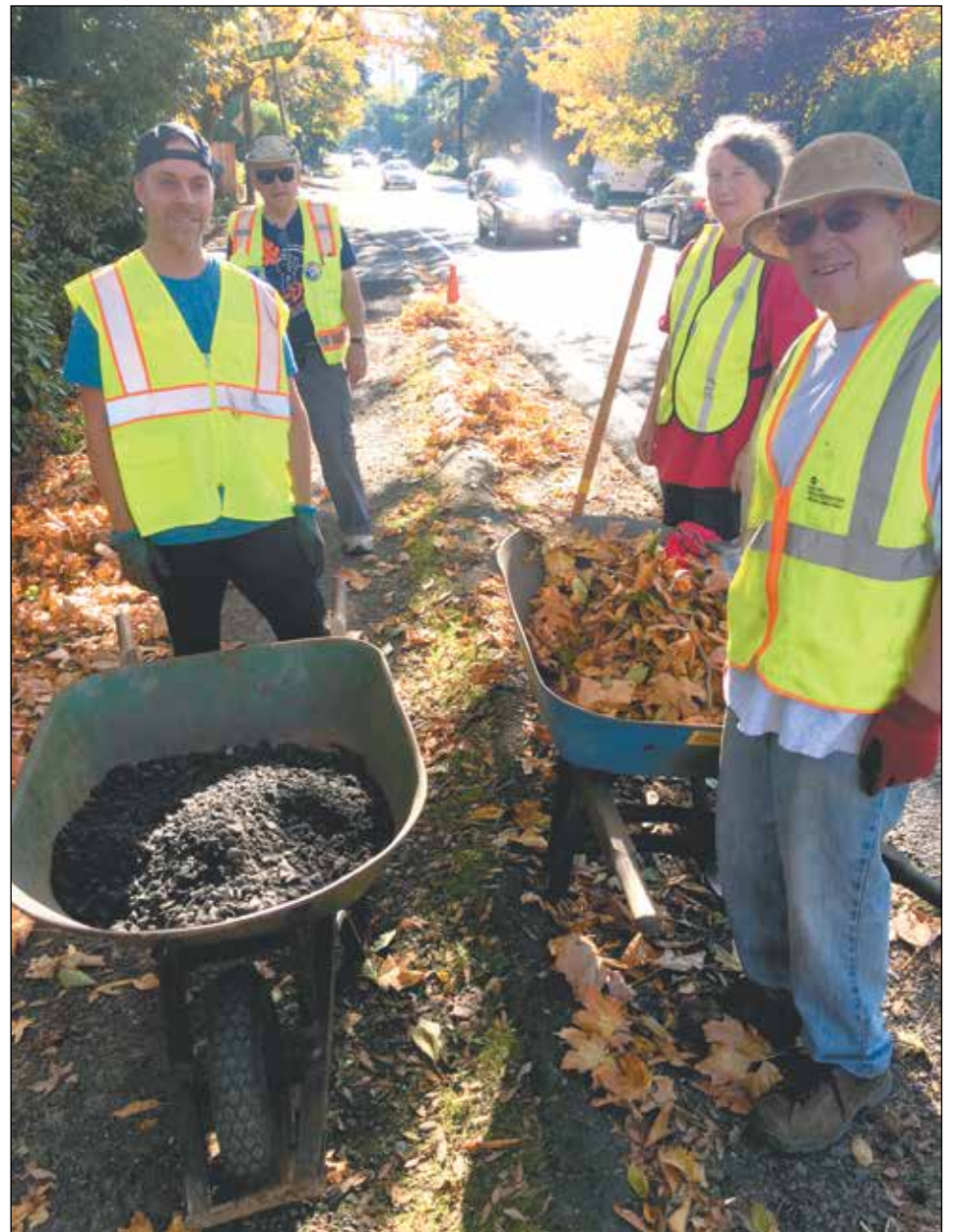
Gravel was delivered by the Portland Bureau of Transportation for the "goat path" along Southwest Capitol Highway on Oct. 28. Volunteers Josh Byler, Donna Jean Paterson, and Chris Houghton use wheelbarrows to spread out the gravel and then tamp it down. Don Baack of SW Trails organized the event. Nearly two dozen neighbors helped out on the brilliant autumn day. (Post photo by Erik Vidstrand)
