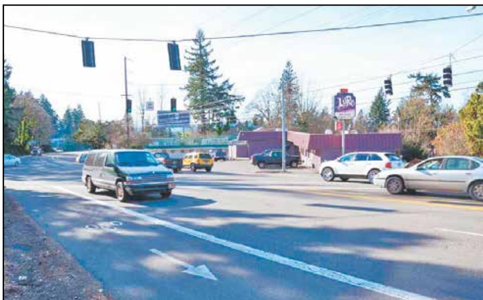
Under a different option, light rail or bus rapid transit could stick to Barbur Boulevard, serving PCC Sylvania from a station here, at Southwest 53rd Avenue. The downside is the 1/3 mile walk to campus. (Photo courtesy of Metro)
