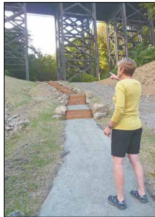
Robin Vesey, Friends of Terwilliger president, points out the new Iowa Street trail, rebuilt by the state, passing under Interstate 5 and Barbur Boulevard viaducts. Grass is growing beside the trail and plants are being added. (Post photo by Janet Goetze)
