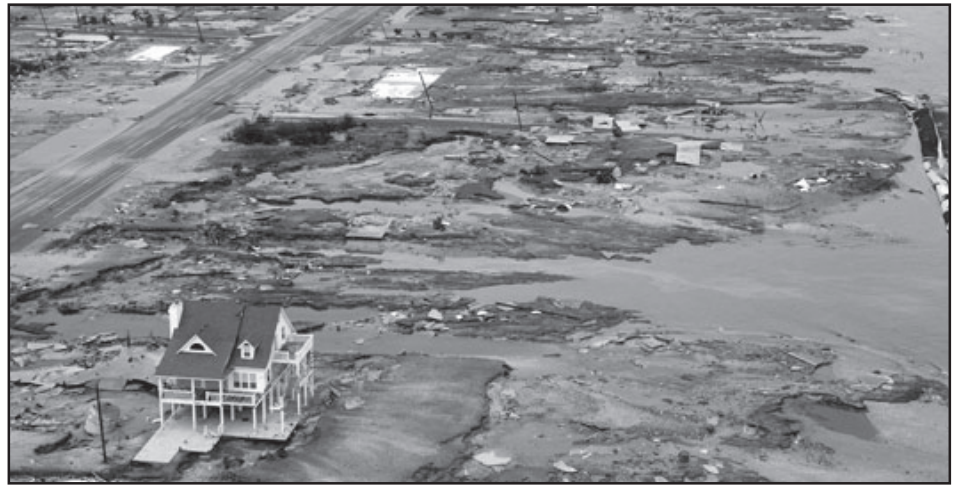
A beachfront home stands among the debris in Gilchrist, Texas on the coast of the Gulf of Mexico on Sunday, Sept. 14, 2008 after Hurricane Ike hit the area. Ike was the first major storm to directly hit a major U.S. metro area since Hurricane Katrina devastated New Orleans in 2005. (Pool Photo/AP)
