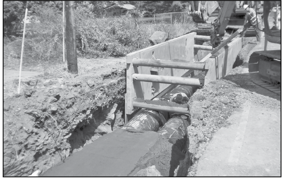
This photo taken July 12, 2010 by a city inspector shows new sewer pipes being installed along Multnomah Boulevard.
