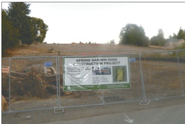
Bare soil and trees gone are among the changes as Spring Garden Park construction continues. (Post photo by Erik Vidstrand)
