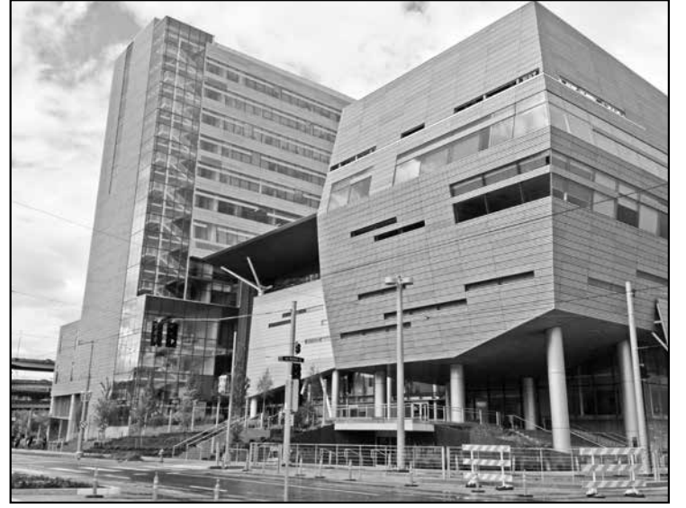
The OHSU Collaborative Life Sciences Building recently opened in South Waterfront. (Post photo by Erik Vidstrand)
