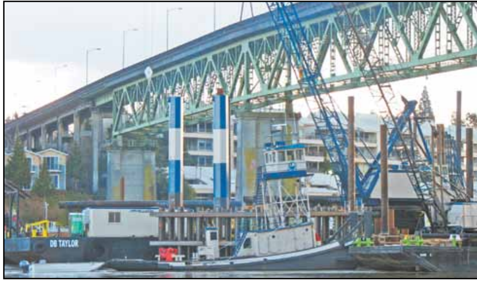
Detour bridge river work being done using a tugboat last month. (Photo courtesy of Mike Pullen, Multnomah County)
