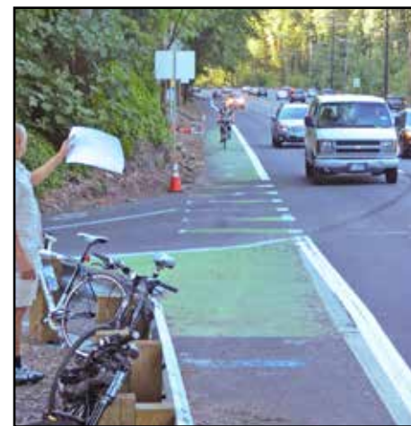
Bicyclists measure and take notes on the thin bike ledge on the Newbury Bridge along Barbur Boulevard. (Post photo by Erik Vidstrand)
