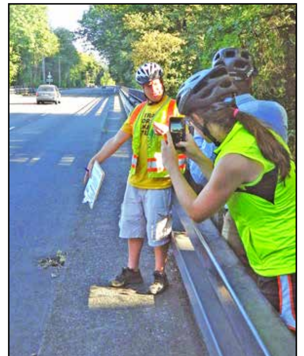
Bicyclists measure and take notes on the thin bike ledge on the Newbury Bridge along Barbur Boulevard. (Post photo by Erik Vidstrand)
