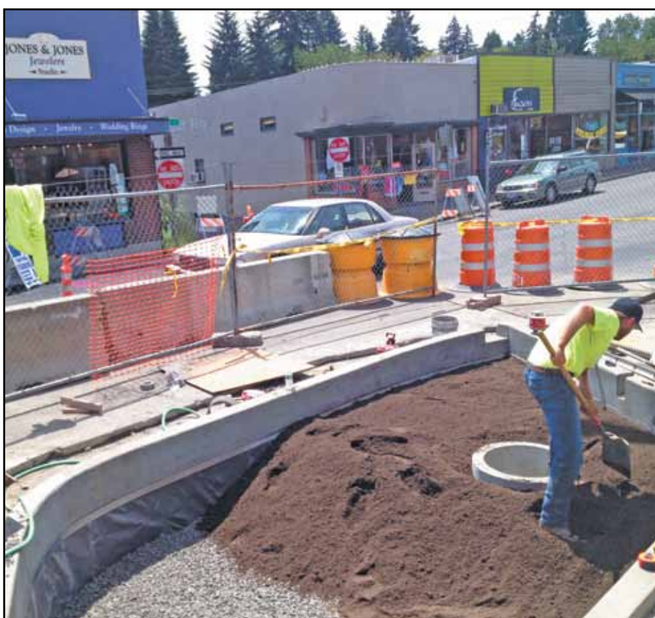
A city contractor works on the new bioswale at Southwest 36th and Capitol Highway in front of ZoomCare. (Post photo by Erik Vidstrand)
