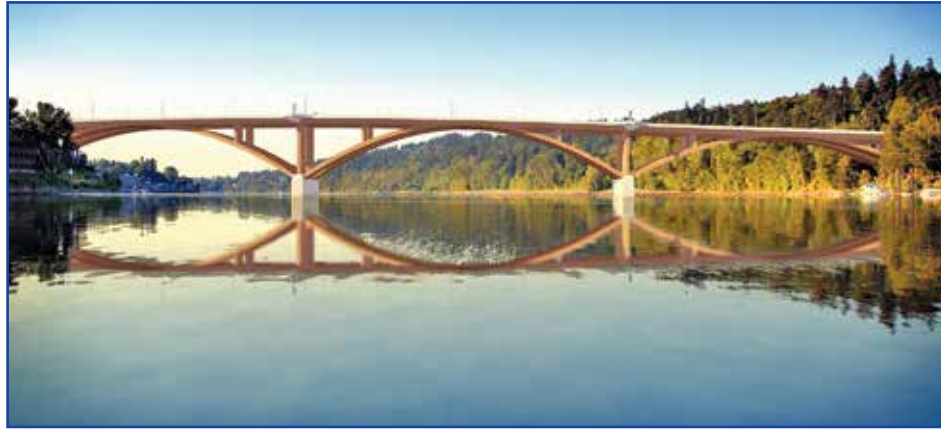
This photo illustration shows the deck arch design of the proposed Sellwood Bridge. (Post file photo courtesy of Multnomah County)
