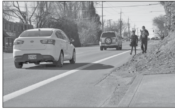
Pedestrians walk along a section of Southwest Barbur Boulevard without sidewalks. The light rail project will be addressing gaps in safe pedestrian routes along the busy corridor. (Photo courtesy of Metro)
