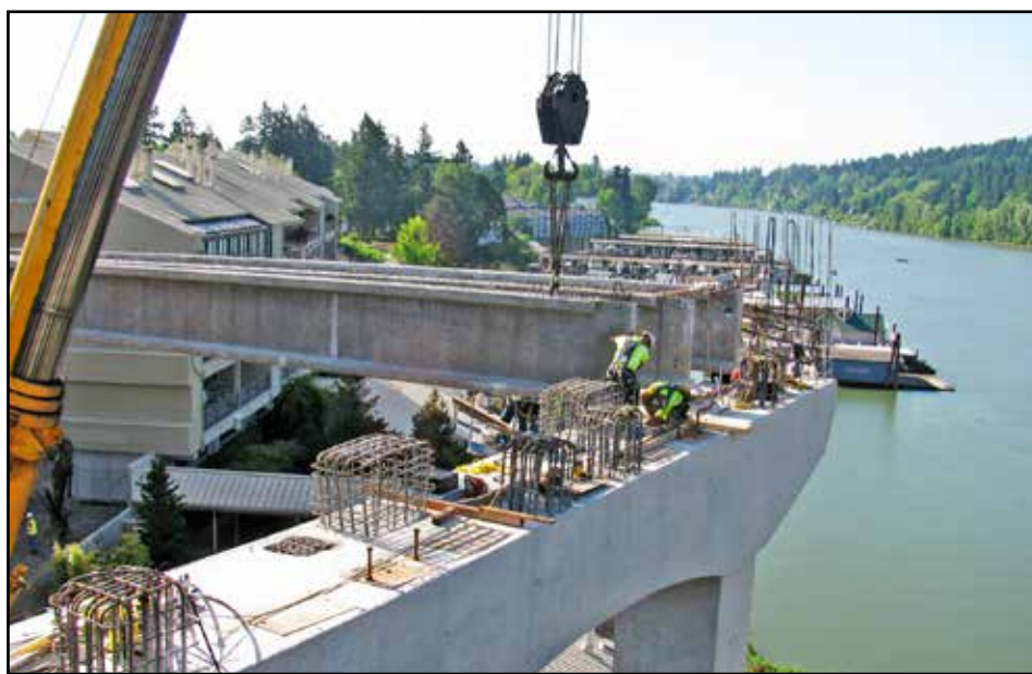
Workers install girders on Bent 6 on the east side approach of the new Sellwood Bridge. (Photo courtesy of Mike Pullen, Multnomah County)
