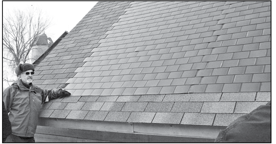
Recently solar shingles have become price-competitive with bolt-on panels, and are getting much more popular accordingly. Pictured: solar shingles from the Dow Powerhouse line. (Photo by Tai Viinikka, courtesy Flickr)
