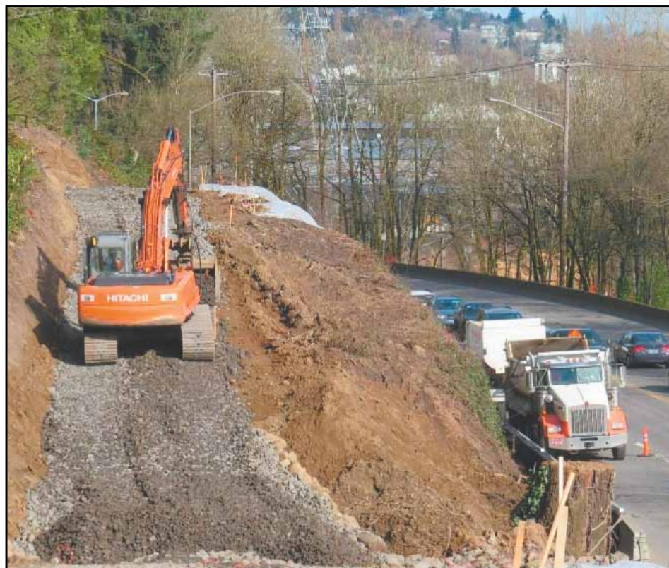
Crews excavate the west side of Highway 43 in preparation for the new Sellwood Bridge. (Photo courtesy of Multnomah County)
