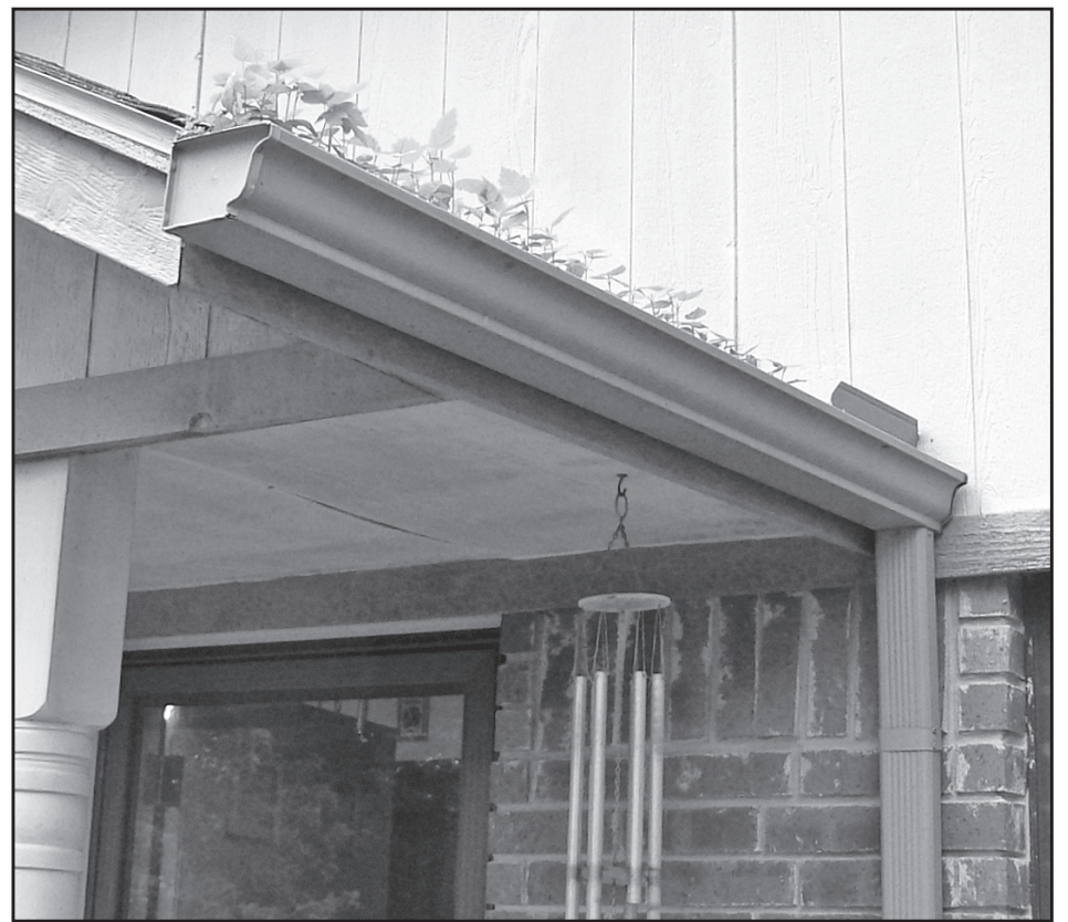
The experts prefer galvanized steel, copper and aluminum gutters for longer life and therefore lower environmental as well as financial cost. Cleaning your gutters now and then is the best environmental option and may preclude any need for replacement. (Photo by Thomas and Dianne Jones, courtesy Flickr)
