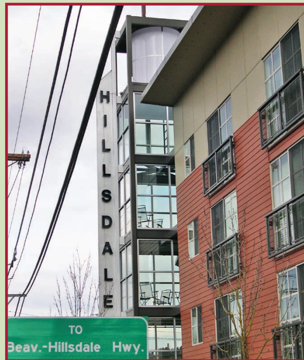
The Hillsdale community raised some $21,000 to help backlight the "Hillsdale" sign on the Watershed building. (Post photo by Don Snedecor)
