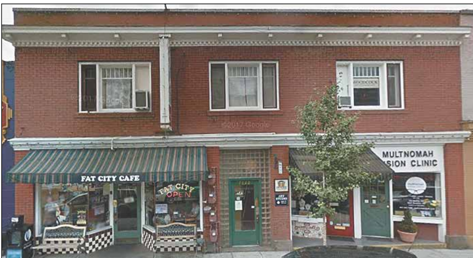
Many of the commercial buildings along Capitol Highway in Multnomah Village are affected by seismic retrofit mandates. (Photo courtesy of Save Portland Buildings)
