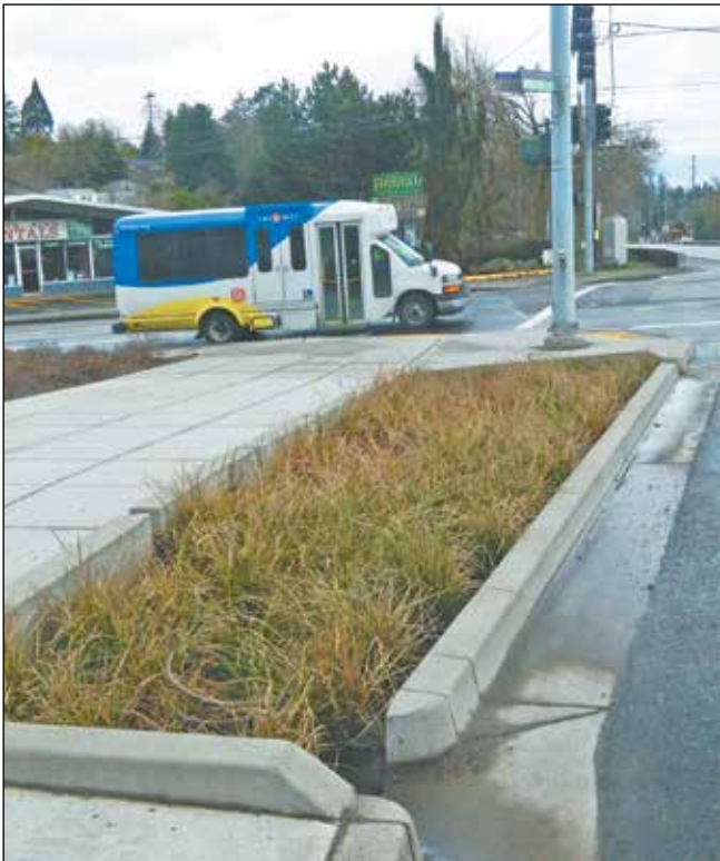
A typical basin bioswale captures water at Southwest Barbur Boulevard and Capitol Hill Road. (Post photo by Erik Vidstrand)
