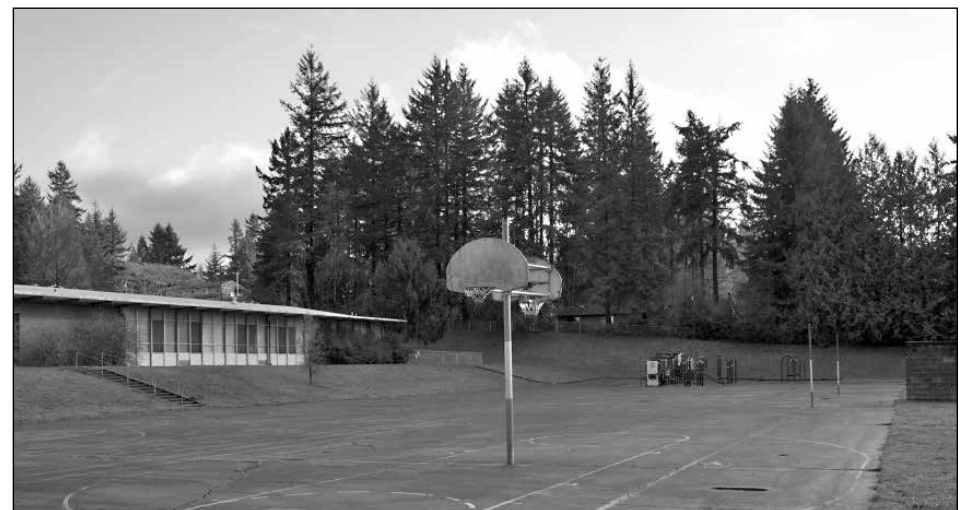
Smith Elementary School closed in 2005 due to declining enrollment and a shrinking district budget. (Photo by Bryan M. Vance, OPB)
