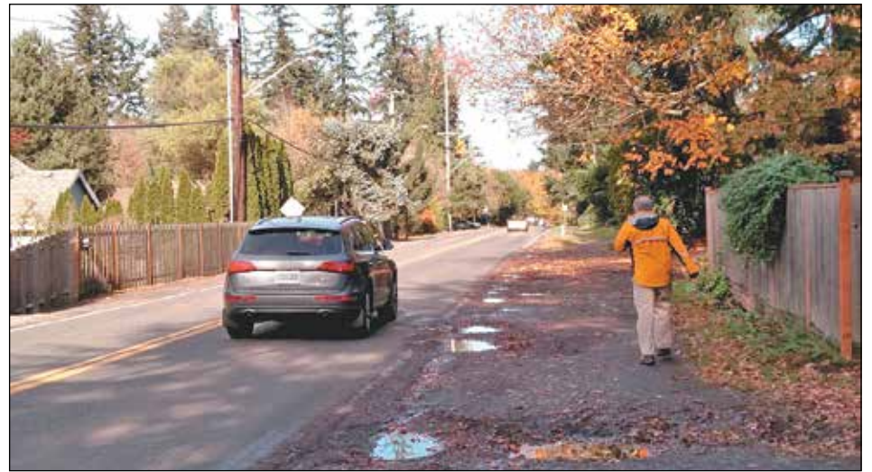
Capitol Highway connects Multnomah Village and the Barbur Transit Center, but lacks sidewalks, bike lanes and stormwater facilities. (Photo courtesy of Portland Bureau of Transportation)
