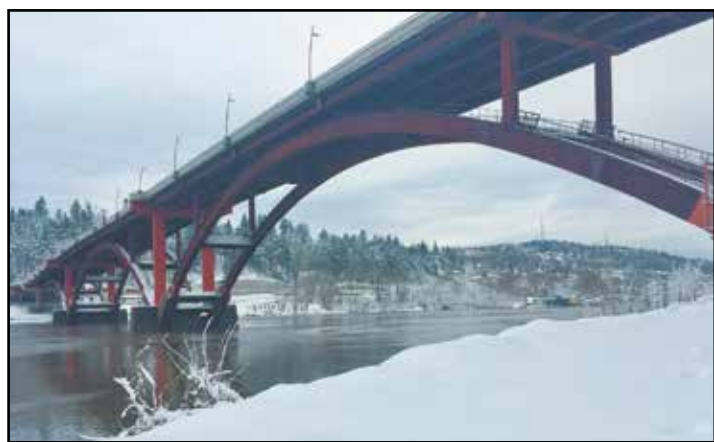
Winter snow covers the new Sellwood Bridge. According to officials the bridge is 99 percent complete. (Photo courtesy of Multnomah County)
