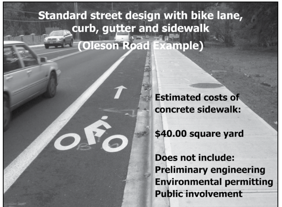
This photo of Oleson Road shows what the north side of Multnomah Boulevard may look like with sidewalks, curbs and bike lanes. (Photo by Roger Averbek)
