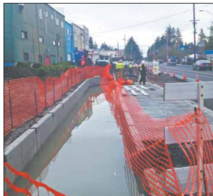
Workers complete construction on a new catch basin and sidewalks along Multnomah Boulevard near 36th Avenue. (Post photo by Erik Vidstrand)
