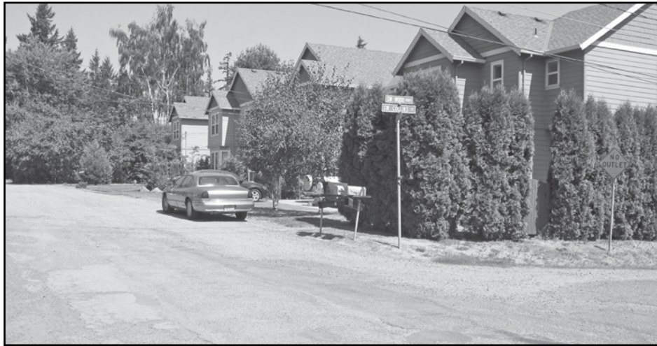
Unpaved street at SW Wood Parkway and Collins St. (Post file photo by Leslie Baird)
