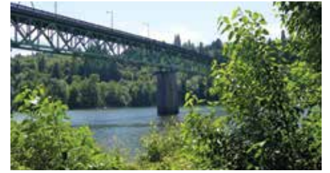
The old Sellwood Bridge as seen from the east bank of the Willamette River in June, 2007. (Post file photo by Don Snedecor)
